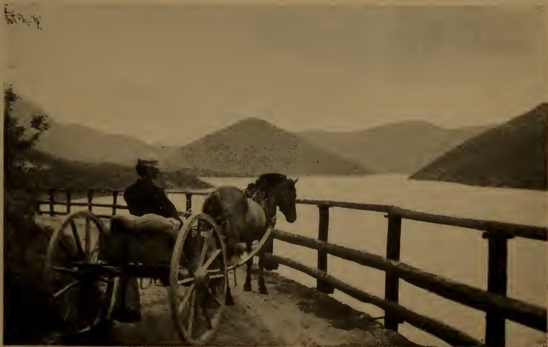
VAAGE LAKE, GUDBRANDSDALEN. The building of this road cost about five dollars a foot.
